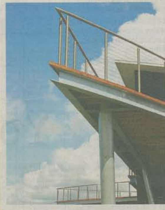
■ Shell Cove Golf Club (BHI): The clubhouse is a key feature of the Shell Cove development and was designed to fit in with its coastal surroundings. The building overlooks the new Shellharbour Links golf course. It is horizontal in shape, excavated into the hillside and appears to be only single storey when viewed from the main approach. Pavilion style roofs are used in the design and a transparent feel exists throughout the building.
