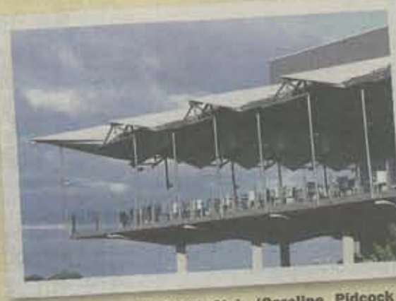
■ Shellharbour Workers' Club (Caroline Pidcock and Richard Goodwin): The roof and balcony extension transforms an existing building to accommodate the need for more space and anticipate future smoking laws. The use of a lightweight steel roof for the new verandah was a logical choice. The roof folds and opens to bring light deep into the balcony area. The new verandah provides external areas for the club for the first time, and will largely be used for outdoor seating for 500 people.
